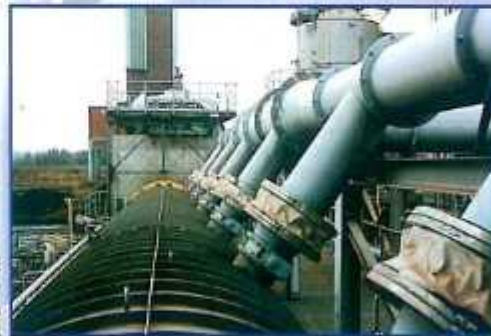
DEKOMTE Joint in the flue gas ducting of a pyrolysis plant
